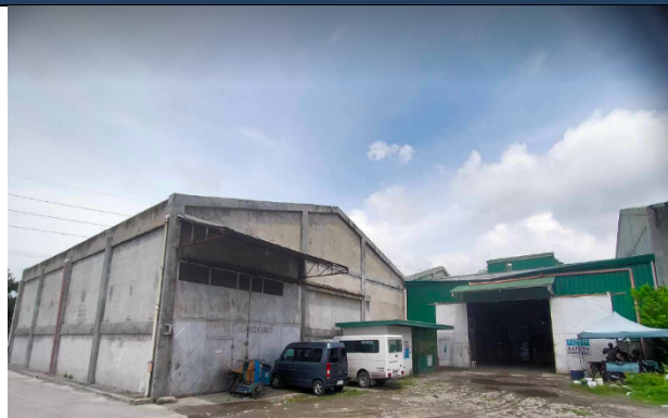
Gensan Plant Façade
