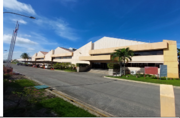
Carmen Plant Façade
